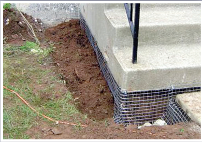
L-Shaped screen application around foundation**
