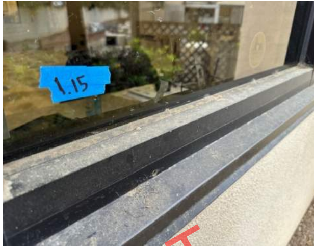
Window 1.15 with weep holes at the sill.
