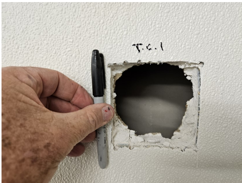
Photograph Number 6 View of relative size of Test Cut No. 1
