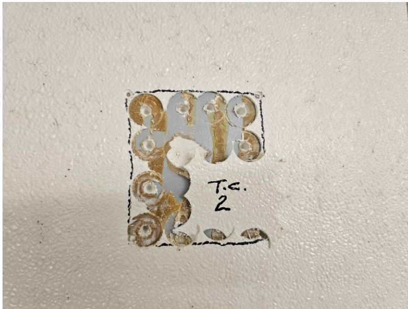
Photograph Number 1 View of FRP & Drywall Behind at Test Cut No. 2
