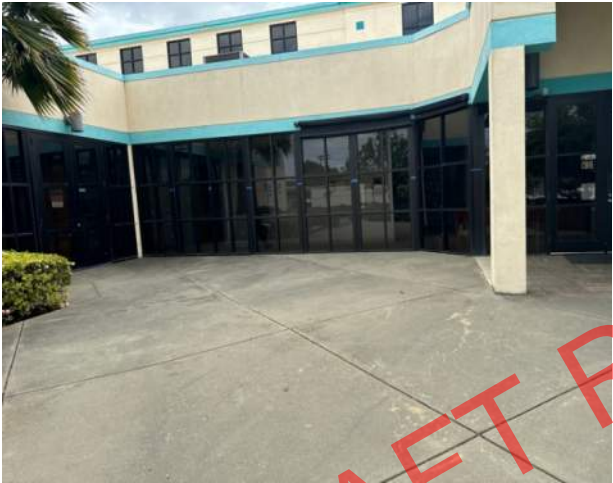
Storefront system at building entry. 4102_NBL01_404
