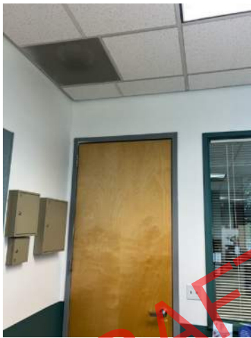
Door to HR Admin Office – door not aligned with jamb. 4102_GEP01_151
