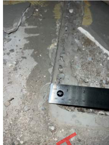
1" sealant joint between new and original slab/footing.
