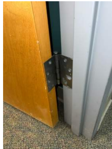
Bottom door hinge seated properly. 4102_GEP01_165
